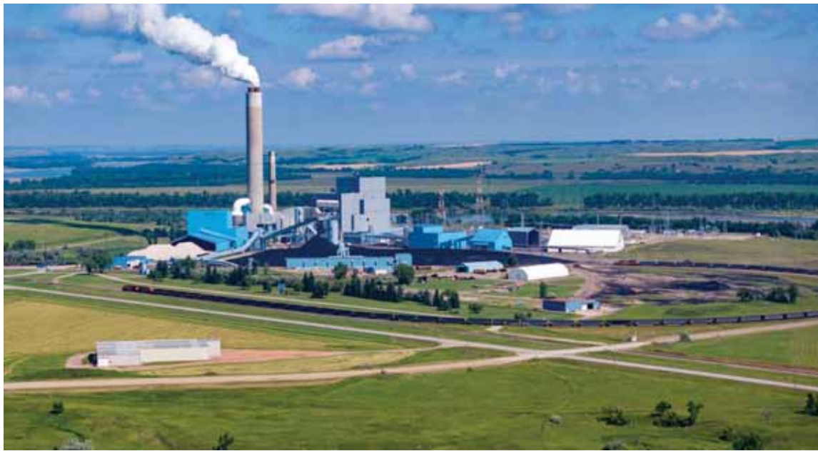
Submitted photo | Jena Gray A view of the Leland Olds Power Plant and surrounding area, including the Missouri River valley in the background.
