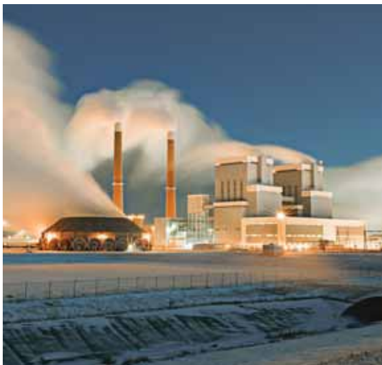
Basin Electric Power Cooperative's Antelope Valley Station provides electricity generation 24 hours a day, 7 days a week.
