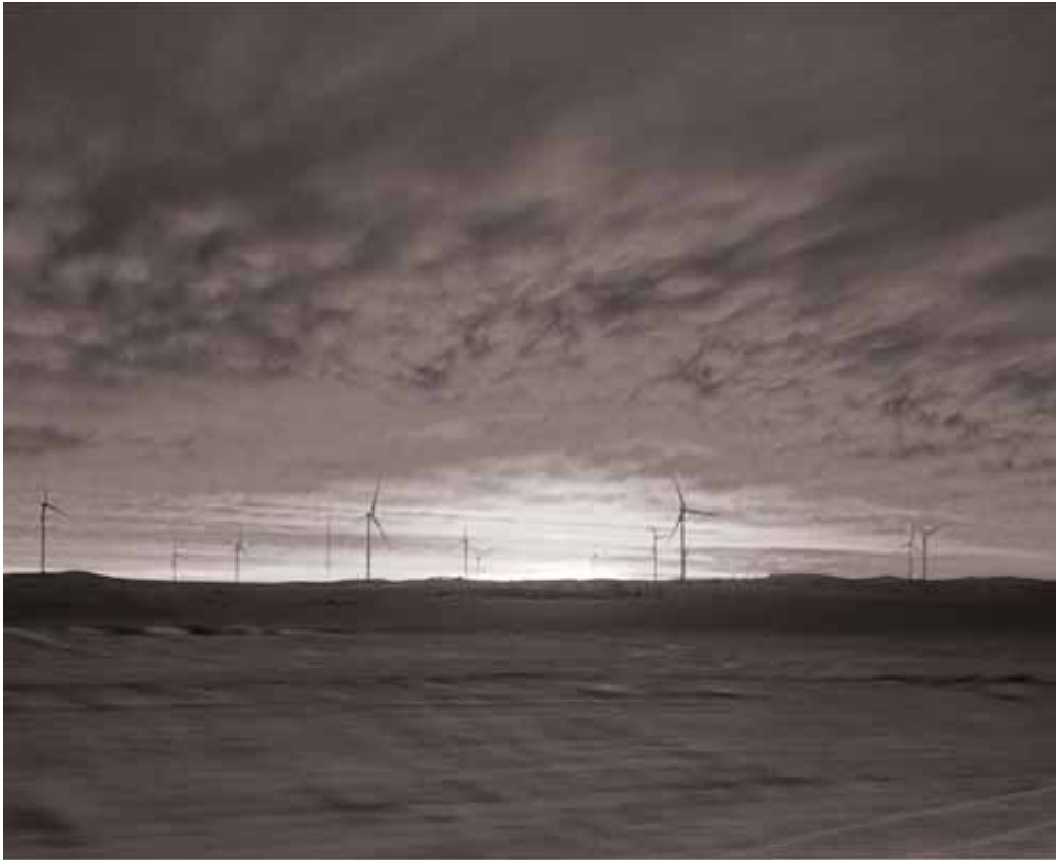
Submitted photo | Mitchell Bettenhausen Turbines silhouetted against a winter prairie sunset, quietly turning wind into power.
