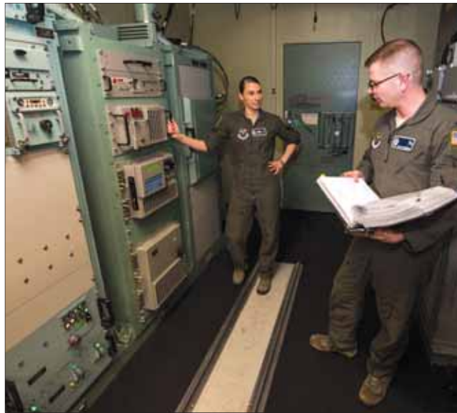
From right, 1st Lt. Alexander Hansen, 742nd Missile Squadron mission lead, and 2nd Lt. Elizabeth Jordan, 742nd MS missileer, go through an inspection at Minot Air Force Base, North Dakota, Jan. 15, 2019. Members of the 742nd MS are responsible for providing day-to-day combat operations for the nation's intercontinental ballistic missile fleet.
