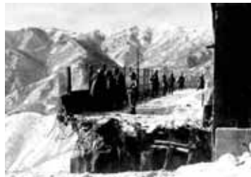
The blown-out bridge at Funchilin Pass. (USAF Photo)
