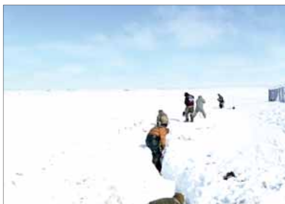
Airmen are shoveling snow April 26, 2022 on Minot Air Force Base, N.D.. They are digging a trench to make sure the launch facility isn't flooded by the melting snow.
