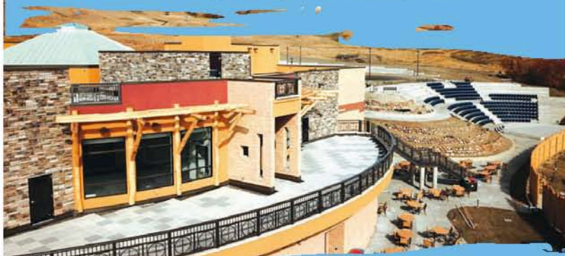
Newly Opened MHA Nation Interpretive Center MHA Nation Interpretive Center Photo
