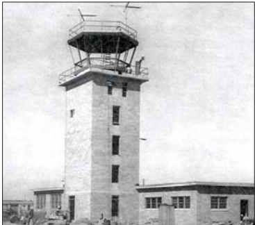
The original base control tower under construction in 1956. (Minot Daily News Photo)
