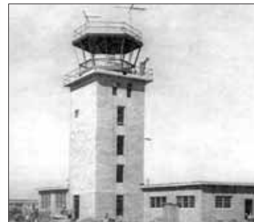
The original base control tower under construction in 1956. (Minot Daily News Photo)
