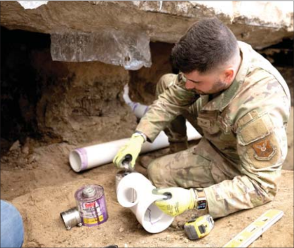
U.S. Air Force Staff Sgt. Darenger Saylor, the 5th Civil Engineer Squadron’s water and fuel systems maintenance non-commissioned officer in charge, prepares polyvinyl chloride pipes inside the hand-excavated command suite of the 5th Bomb Wing headquarters on Minot Air Force Base, North Dakota, April 16, 2025. Members of the 5th CES excavated the exterior trench to access a manhole so the old cast-iron pipes could be replaced with modern PVC pipes.
