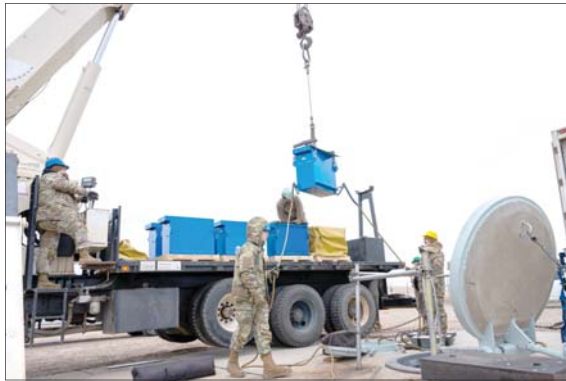
Airmen from the 91st Missile Maintenance Squadron's electro-mechanical team (EMT) guide a replacement battery into a launch facility near Minot Air Force Base, North Dakota, April 2, 2026. A significant portion of EMT's work involves "remove and replace" procedures, in which aging or worn components are swapped out before they fail.
