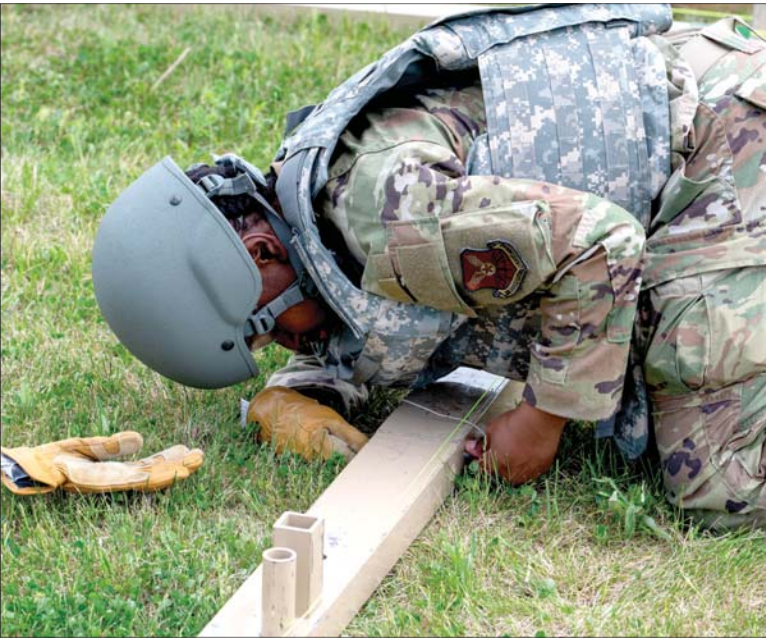
U.S. Air Force Airman 1st Class Alannique Jacobs, assigned to structures, 5th Civil Engineering Squadron builds the baseboards for a medium California tent during the bivouac exercise at Fargo Air National Guard Base, North Dakota, May 31, 2026. Medium California tents are capable of housing large assets, serving as a maintenance bay, or operating as a command center in extreme climates.
