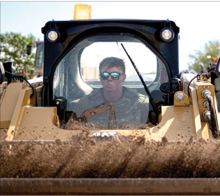
Senior Airman Mathew Plummer, pavements and equipment journeyman, 5th Civil Engineering squadron operates a compact tract loader, while repairing a crater during the bivouac exercise at Fargo Air National Guard Base, North Dakota, June 2nd, 2026. The objective of the crater repair exercise is to rapidly fix bombed-out runways so aircraft can continue to land and launch under pressure.
