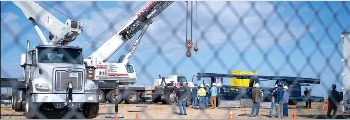
Missile maintenance technicians assigned to the 583rd Missile Maintenance Squadron prepare to lift a missile suspension system with a crane at a launch facility near Minot Air Force Base, North Dakota, Aug. 18, 2026. The 583 MMXS is responsible for the routine and preventative maintenance of launch facilities across the Department of War, ensuring nuclear deterrence capabilities remain safe, secure, reliable, and ready to respond at a moment’s notice.
