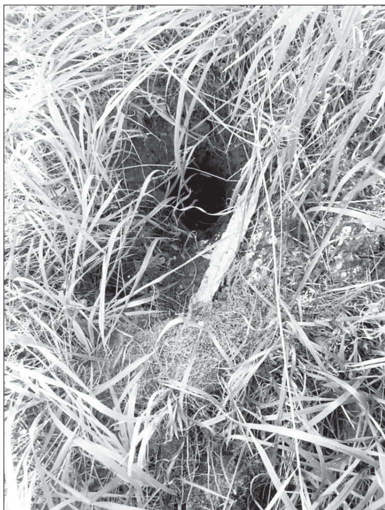
The end of the metal legs grounded the structure and 16-inch holes in the soil were the result of the lightning reaching the bottom of the stand.
