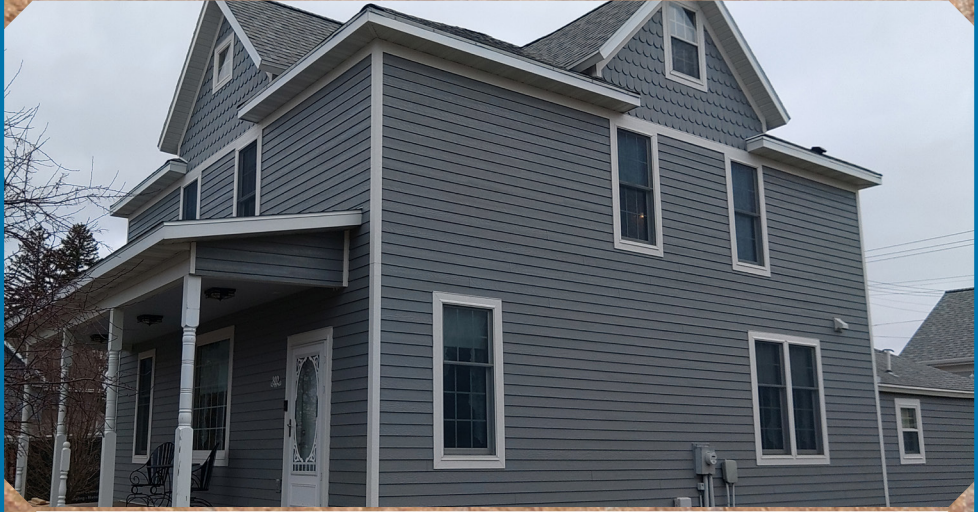
Residing Project with DiamondKote LP Smartside with decorative scallops ungable ends
