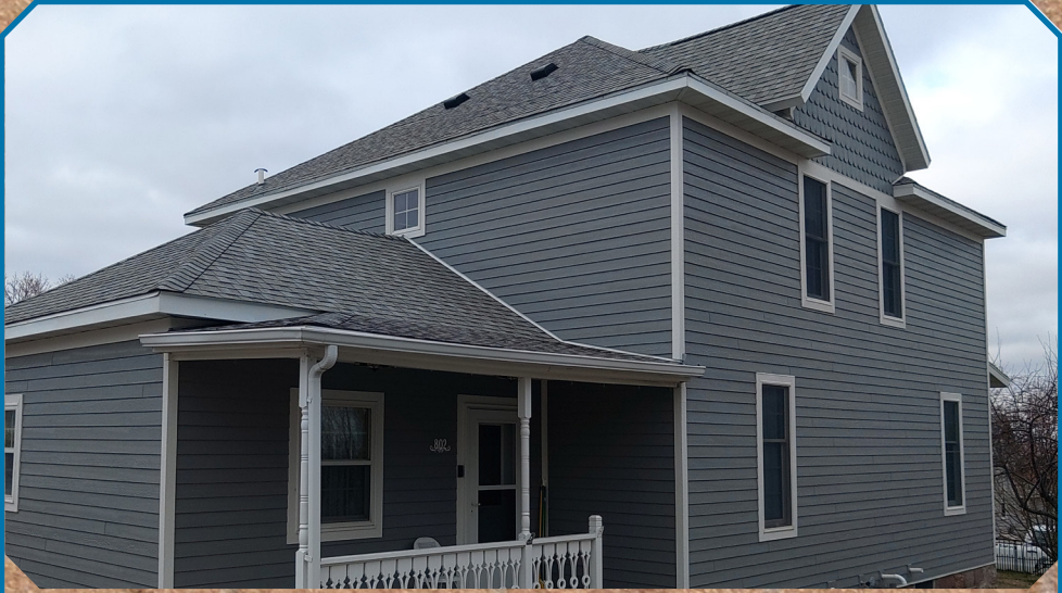
House Remodeling project CertainTeed asphalt shingles, Mastic Steel siding and Versetta on dormers/garage
